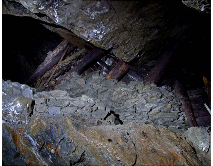
New supports for sagging timbers in Cwmystwyth
