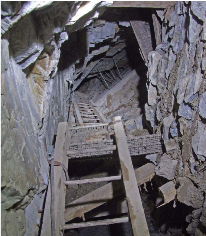
Refurbished shaft in Talybont
