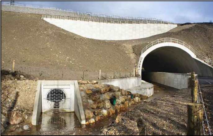
Carno Adit (grilled) with the new A470 running above
