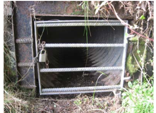
The level 3 entrance portal
